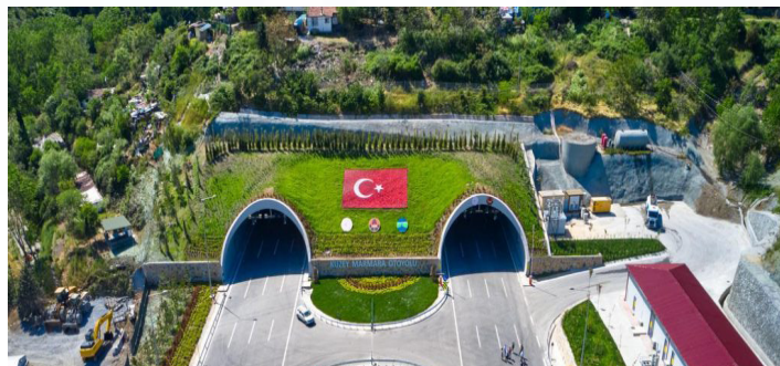
North Marmara Highway
